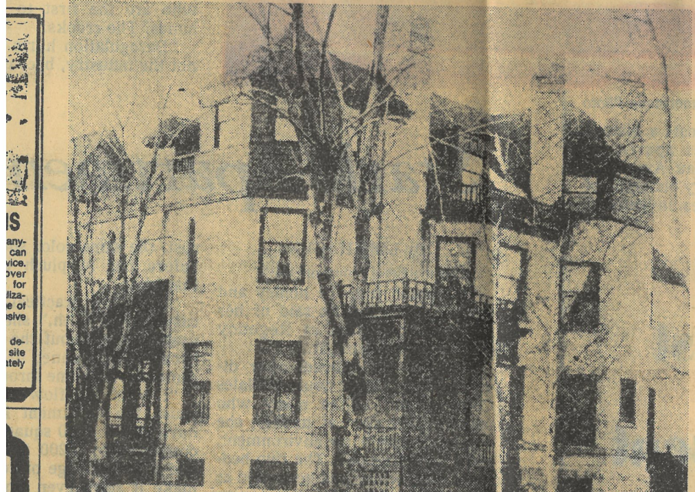
This photo of the Henry L. Palmer house, 1042 E. Juneau, is from an old souvenir book published by the Evening Wisconsin in 1891. A comparison of chimneys and the bay leads architectural historian H. Russell Zimmermann to suspect that the house actually encases the original C. Latham Sholes
